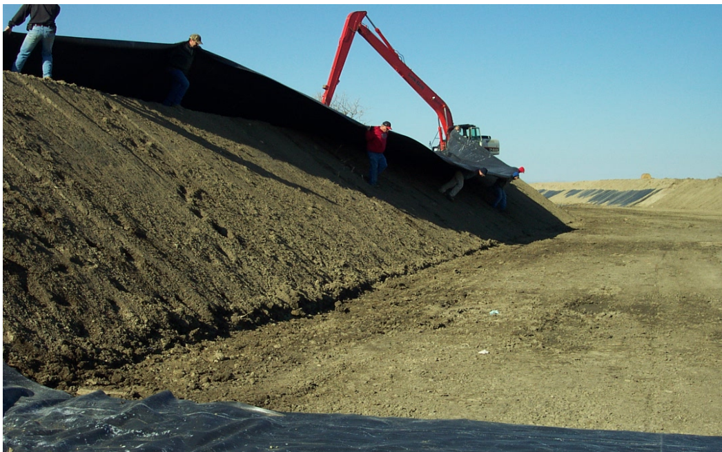
Figure 3-5. Lining of the Inlet Canal.
