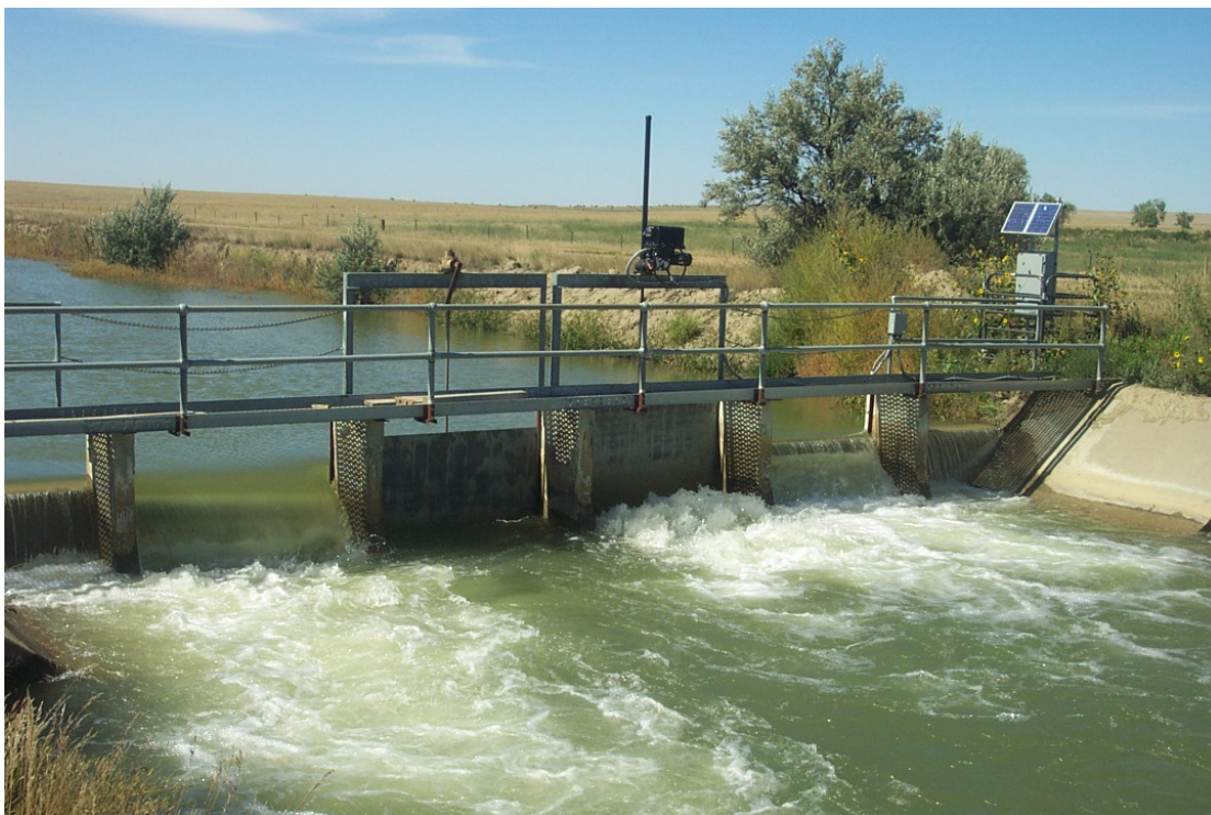
Figure 3-2. Gate Automation Unit Installed in the Belle Fourche Irrigation District.
