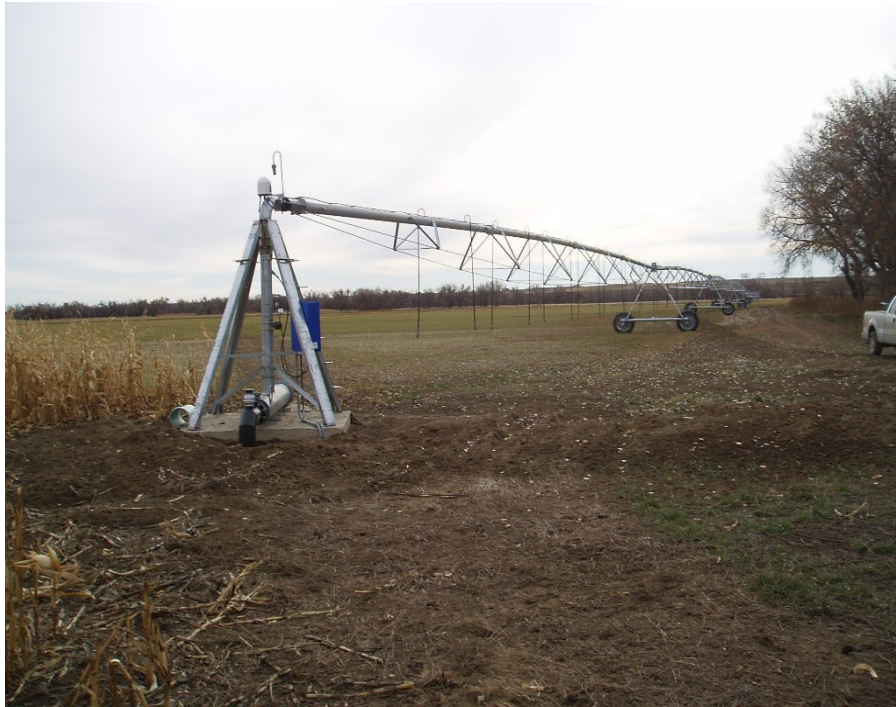
Figure 3-3. Center Pivot Installed in the Belle Fourche Irrigation District.
