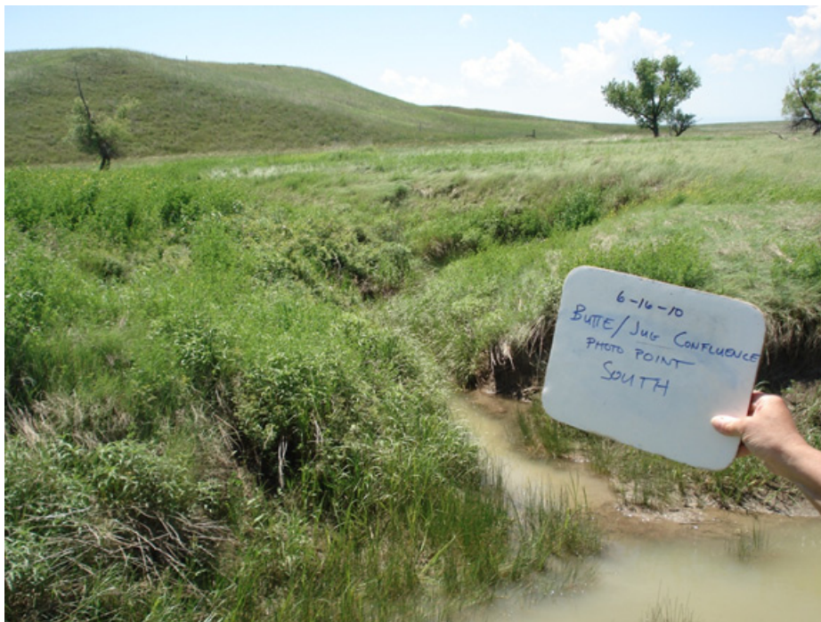
Figure 3-8. Photograph Monitoring Site After Planned Grazing Best Management Practice Installation in 2010.
